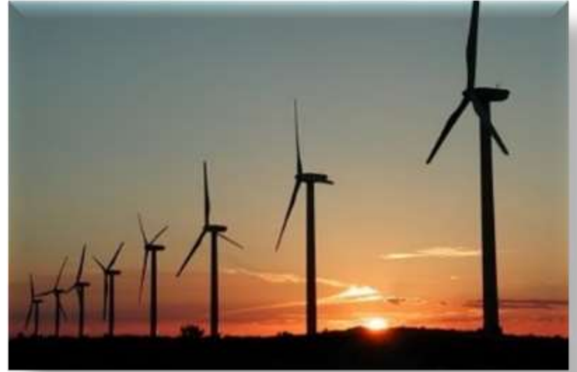
Zaafarana Wind Station, Egypt
